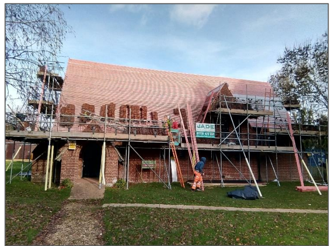
Our roof is being thoroughly refurbished
